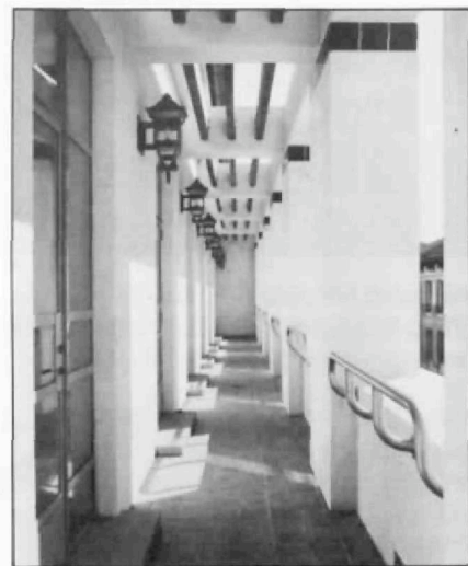
Second-floor corridor, Goldsmith Hall.
