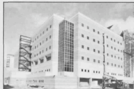
Ben Taub Hospital, CRS Serrine and Llewelyn-Davies Sahni, to be completed in 1989. Ben Taub, one of two large hospitals operated by the Harris County Hospital District for patients unable to afford private care, is in fact one of the most handsome of the new structures under construction. The alternating brick bands take their cue from Cesar Pelli's work at Rice University, and the glazed stair towers offer the promise of orientation from inside the building. The original 1963 building will be taken over by Baylor.
