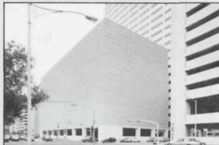
Smith Tower, Lloyd Jones Fillpot & Associates, 1988. Methodist was also the client (with Century Development Corporation as developer) for this smooth-skinned 25-story tower across Fannin, notable especially for the elegance of its parking structure, which has two ramps spiraling in opposite directions at its base and beautifully taut aluminum slats drawn in horizontal patterns across its ten-story volume. The stodgy interiors of the tower are peculiarly incongruous with the no-nonsense exterior.
