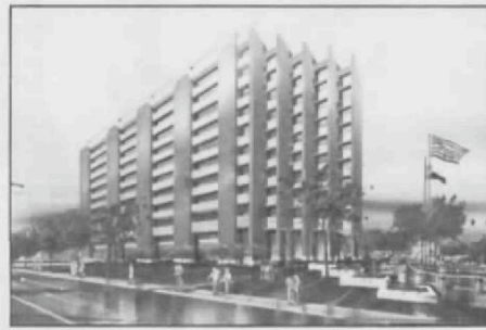
Texas A & M University Institute of Biosciences and Technology, Bernard Johnson, to be completed in 1990. The first of two 11-story laboratory buildings, of concrete frame with brick veneer and designed according to the regimented taste of its client to be almost without character, will be built this year on the site of the Shamrock swimming pool. A "water feature" is being planned by the TMC (with funding from the Wortham Foundation) to liven up the Main Street tip of the triangular site.
