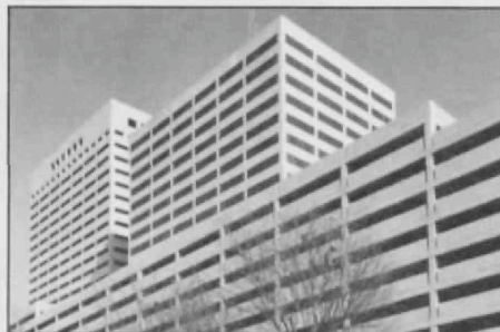
Scurlock Tower, S. I. Morris Associates, 1980. Methodist was again the client (with Gerald D. Hines as developer) for this earlier and less well proportioned twin of Smith Tower. Black aerial tubes link Scurlock to Smith and both towers to the hospital complex. Scurlock's fourth floor houses the Sid Richardson Institute for Preventive Medicine, comprising both Chez Eddy (a restaurant named after oil-magnate donor Eddy Scurlock that serves a gourmet menu approved by the American Heart Association) and a health club with indoor track whose exuberant Postmodern interior, designed by William T. Cannady & Associates, inverts the tendency to dress up the façade.
