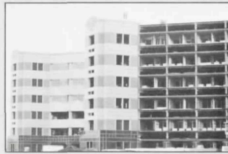
Veterans Administration Medical Center, 3D/International and Stone Marracini and Patterson, to be completed in 1989. This will be the largest and most innovative hospital of the new crop. With utilities floors sandwiched between the working floors, it will allow alterations to be made to the mechanical system without interrupting service. The plan, which from the exterior appears complex due to the shifted orientation of the corner towers and the jogging configuration of the bays, is actually based on a simple long corridor spine, 16 feet wide, running diagonally through the center of the building.
