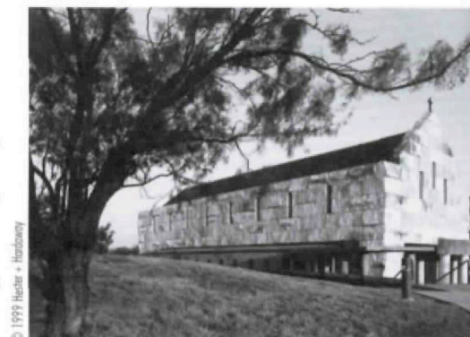
© 1999 Heister + Hardaway Side and front facade, Cistercian Abbey Church. A 13th-century church in Hungary provided a model for Cunningham's use of light and dark stones.
