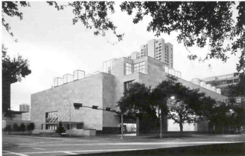
During the day, the lanterns atop the Beck Building capture light for the galleries. In the evening, they glow.
