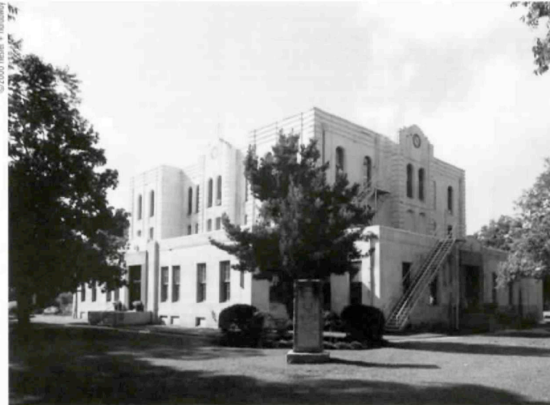
The Wharton County Courthouse as it is: A recent photograph shows the Art Deco remodeling from 19
