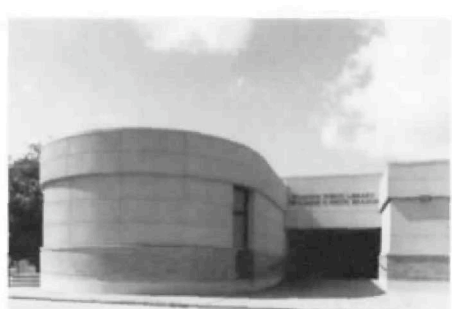
Smith Branch , 3624 Scott Street, John S. Chase, 1974; renovation, Ziegler Cooper, 2001.
