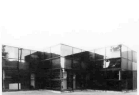
Carnegie Branch , 1050 Quitman, Ray Bailey Architects, 1982.
