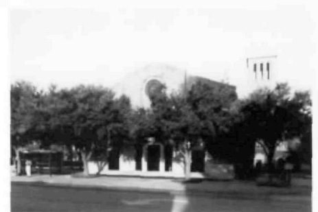
Freed-Montrose Branch , 4100 Montrose, conversion of William Ward Watkin's 1941 Central Church of Christ, Ray Bailey Architects, 1988.
