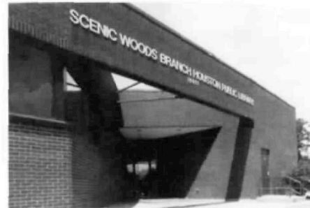
Scenic Woods Regional Branch , 10677 Homestead Road, James. L. Marshall Associates, 1986
