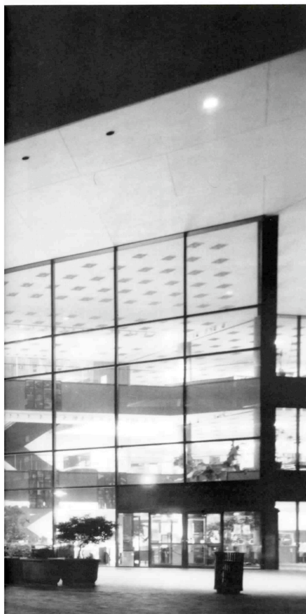
The Jesse H. Jones Building, designed by S.I. Morris Associates and opened in 1976, has served as the Houston Public Library's central branch for a quarter of a century. But it may no longer be up to the job.
