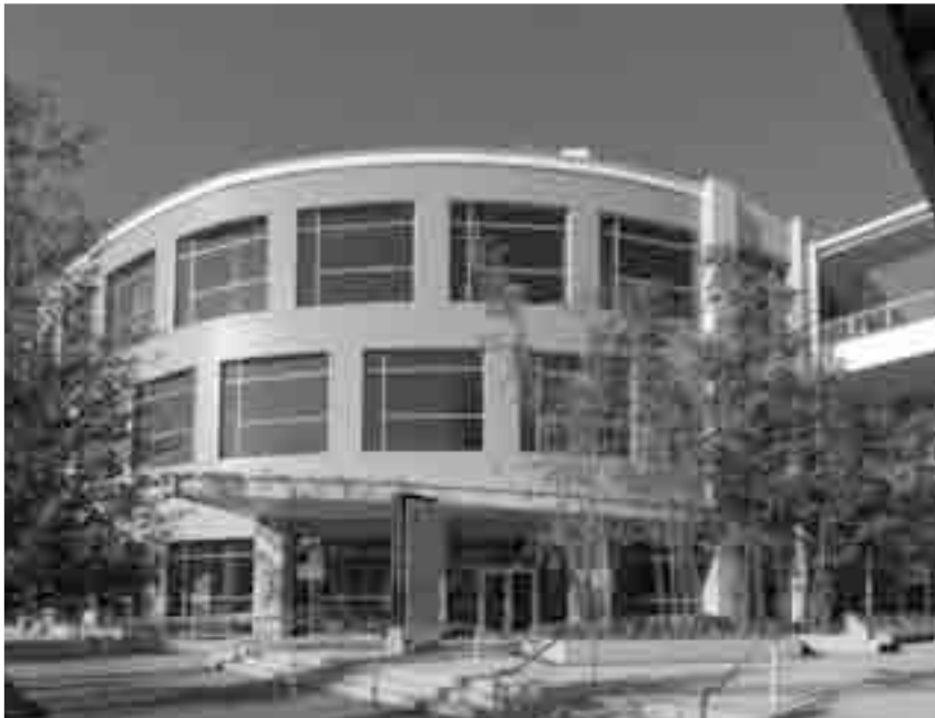
The entrances on the east and west sides of the Houston Pavilions feature lively and inviting façades.
