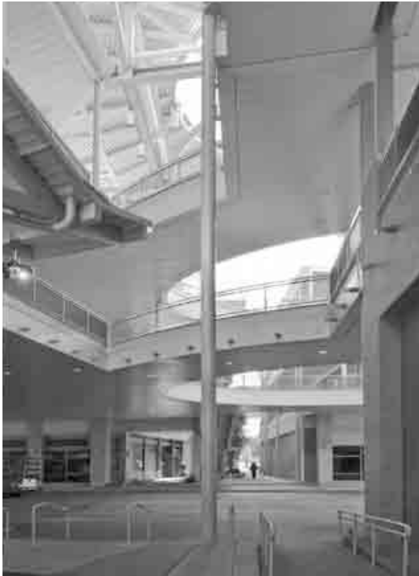
The ground floor of the central spine lacks crossings at Fannin and San Jacinto.
