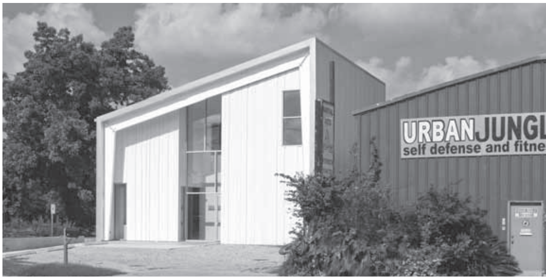
Front façade showing pre-engineered structure and vertical siding.
