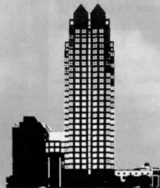
SUN BANK CENTER Orlando, Florida Skidmore Owings & Merrill
