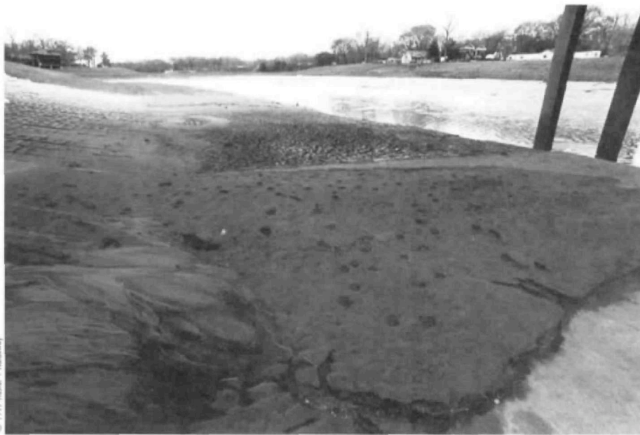
Simms Bayou at Broadway, laid back to prevent flooding and allow natural vegetation to reestablish itself.
