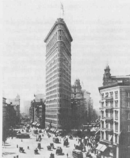
The Flatiron Building, 1903, Daniel H. Burnham and Company, architect (Photo courtesy New York Historical Society)
