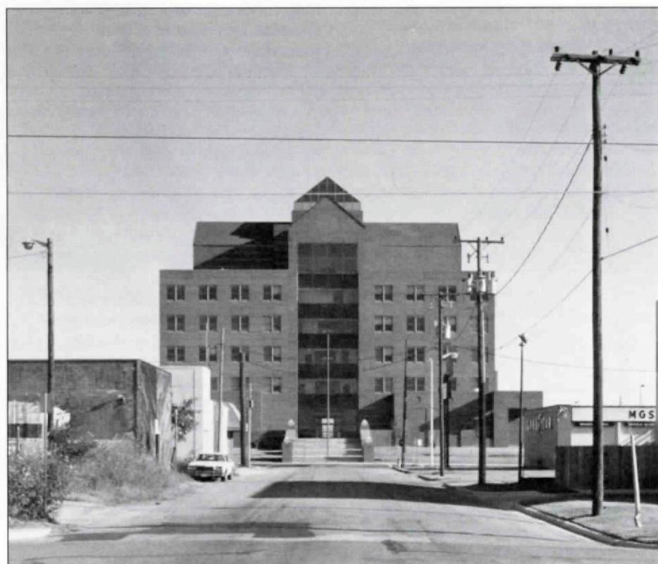
North façade, Corpus Christi City Hall.
