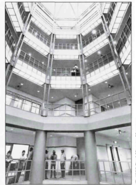
Labroustean use of metal members for the interior balconies, Corpus Christi City Hall.
