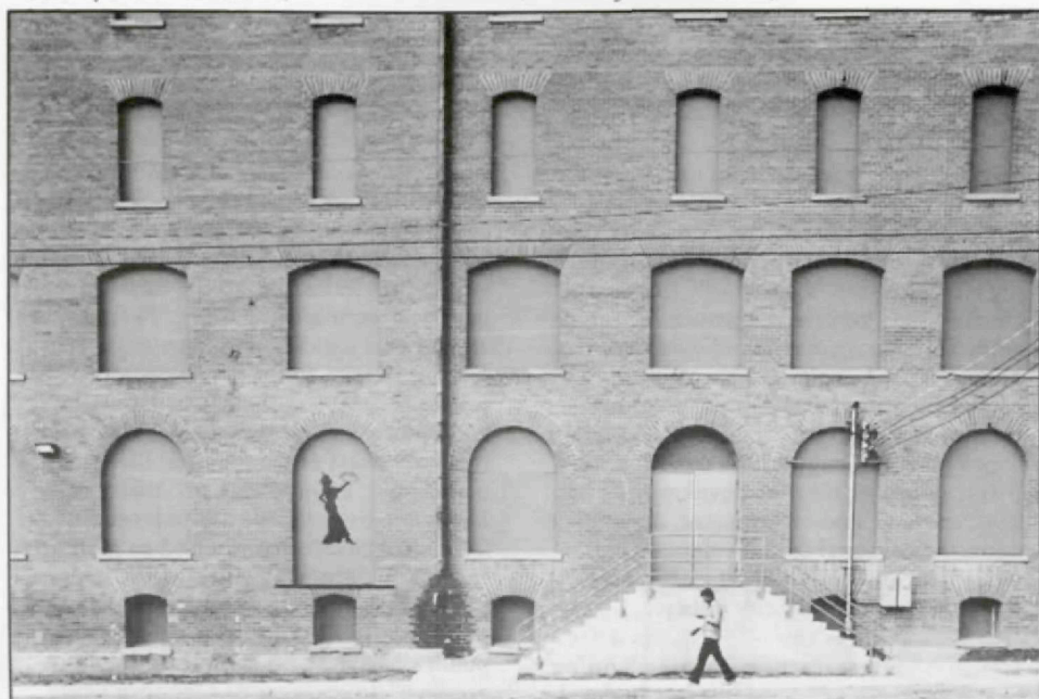
Detail of south elevation, El Mercado del Sol (Photo by Paul Hester)
