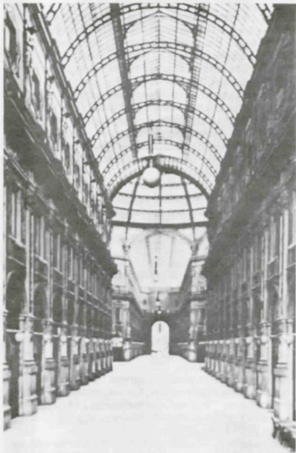
Galleria Vittorio Emanuele, Milan, 1865-1877, Giuseppe Mengoni, architect (Architecture: Nineteenth and Twentieth Centuries, Baltimore, Penguin Books, 1958)
