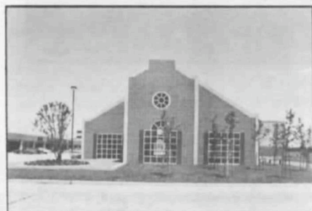
Dairy Ashford Village, Dairy Ashford (Photo by Paul Hester)
