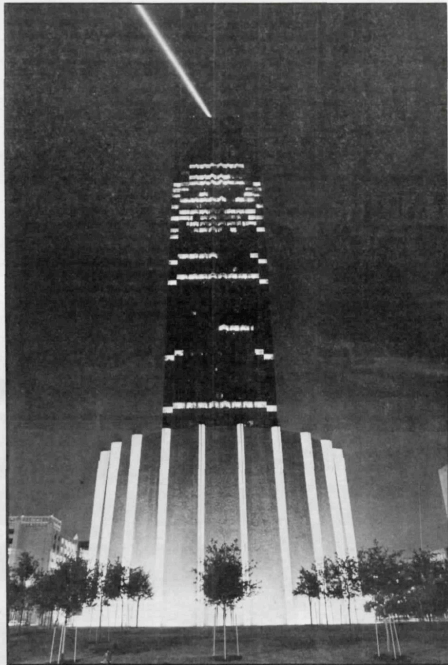
Rear elevation, the Transco Fountain (Photo by Paul Hester)
