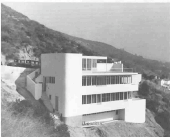
Kun House, 1936, Los Angeles. Richard Neutra, architect.
