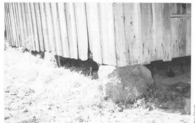
Barn 1, ironstone footing.
