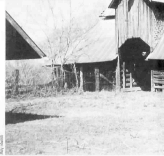
Barn 2, looking northeast.
