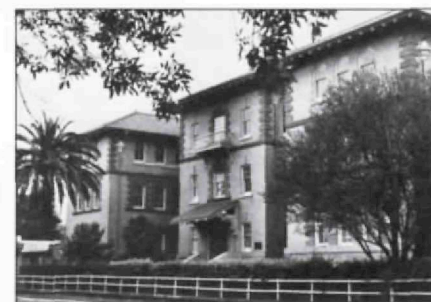
Southern Pacific Railroad hospital, Department of Building and Bridges, G.H.&S.A. Railway, architects, 1911. Thomas Street Center renovation, 1989.
