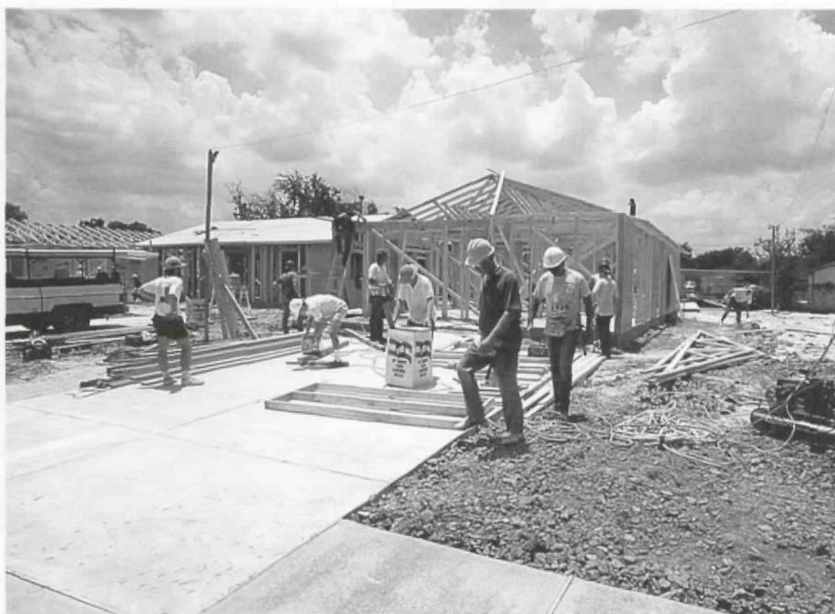
House raising, Habitat for Humanity, Houston chapter.
