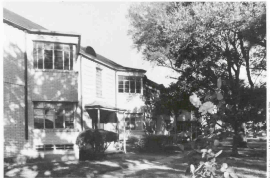
Daniel Armstrong (Eugene Werlein, architect of record), Wilshire Village Apartments, 1940. View along Dunlavy Street.
