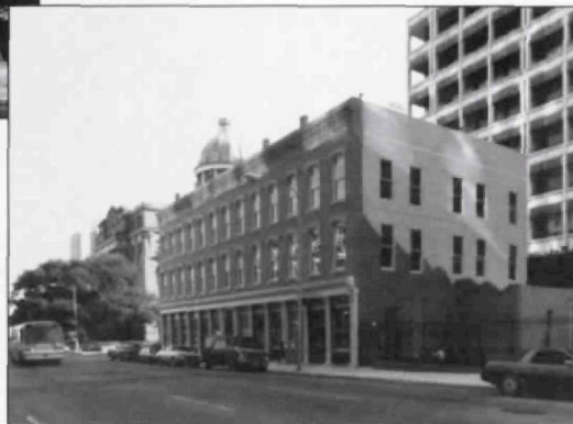
Above: The Pillot Building in 1983. Right: Pillot Building reconstruction, 1990, Morris Architects with Barry Moore, restoration architect. Only the cast-iron architectural elements of the 1860 building remain in place.
