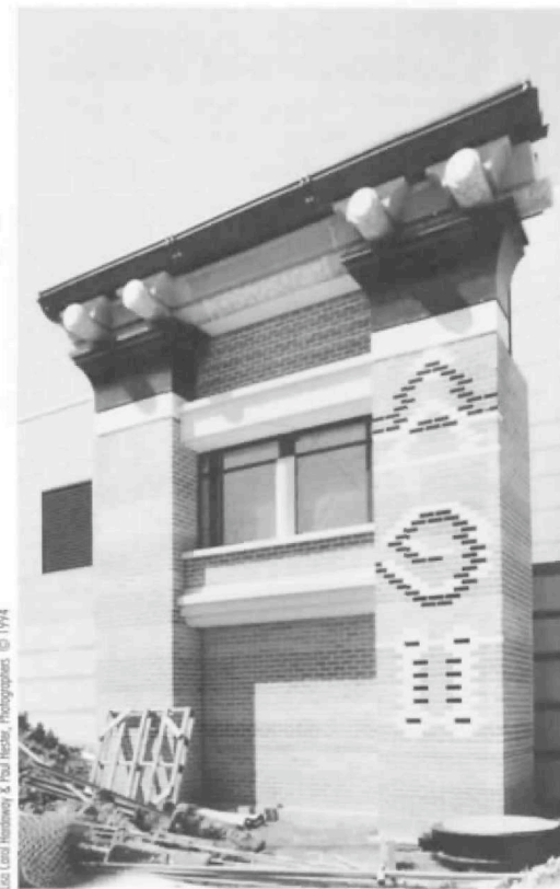
Mockup of partial wall section showing skin treatment and pseudo-Chinese bracketed rafters.
