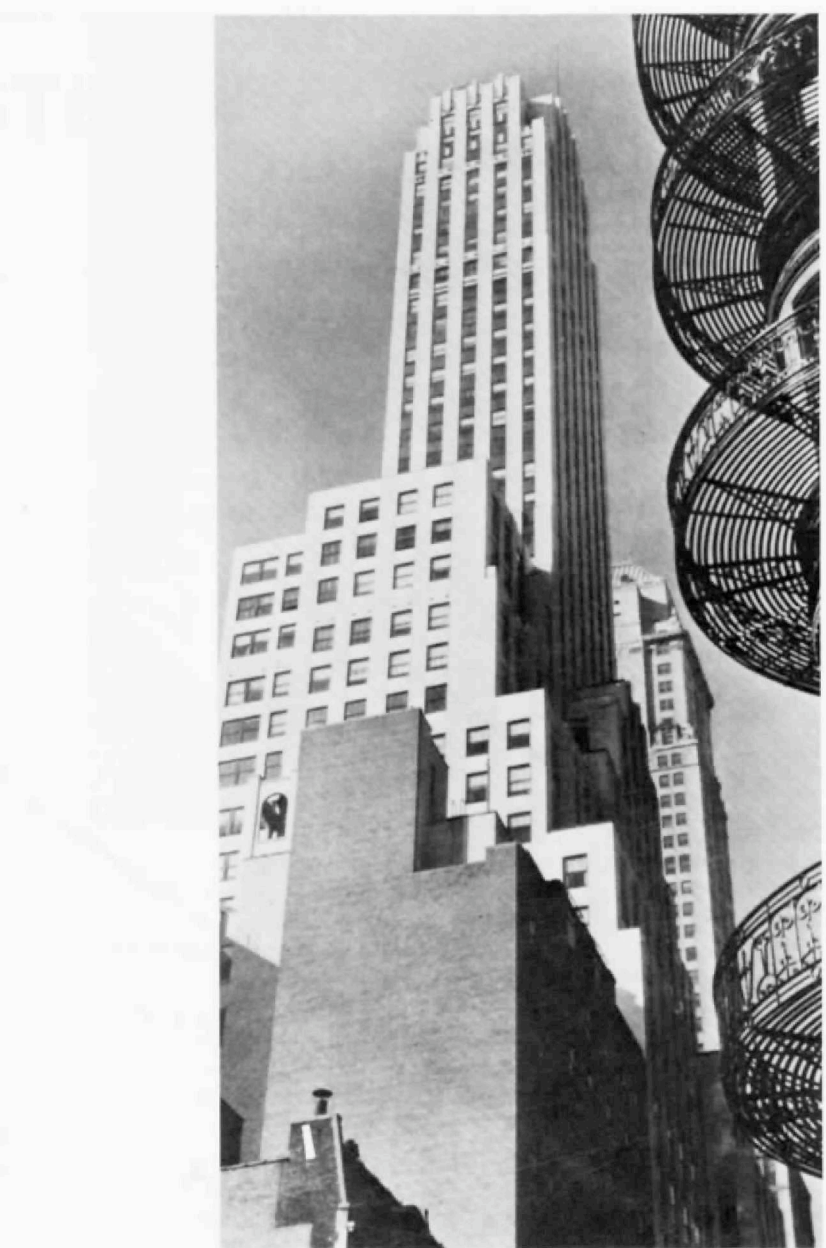
22 East Fortieth Street, 1931, Kenneth Franzheim
