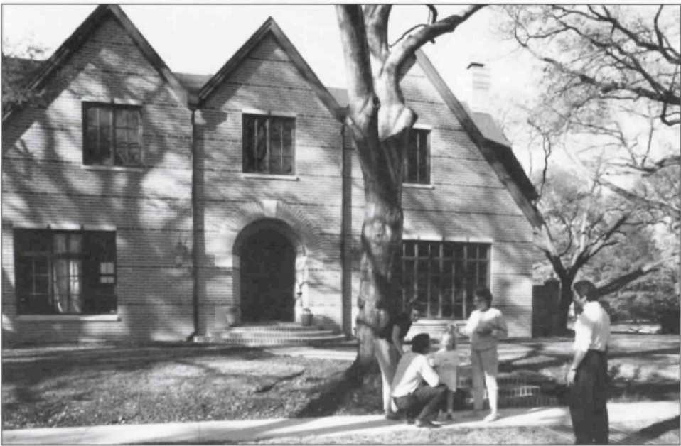
Ziegler House, 1990, Ziegler Cooper Architects, front elevation.
