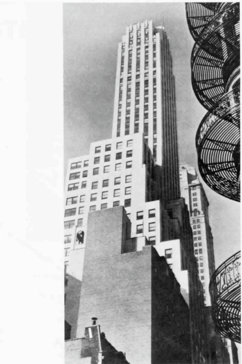
22 East Fortieth Street, 1931, Kenneth Franzheim
