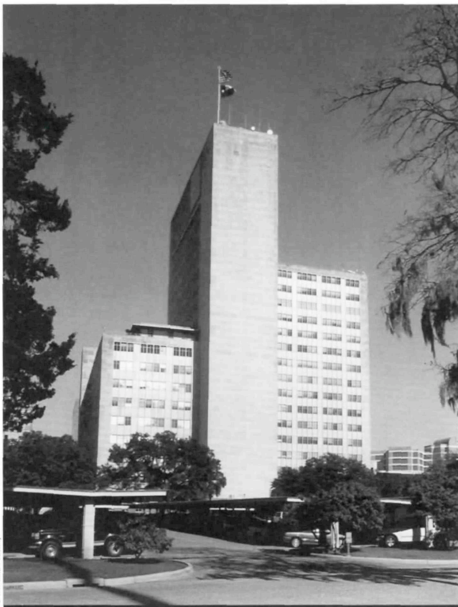
Prudential Building, 1100 Holcombe Boulevard, Kenneth Franzheim, architect, 1952.
