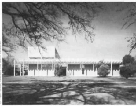
© Paul Henze, courtesy The Menil Collection The Menil Collection, 1515 Sul Ross, Renzo Piano architect with Richard Fitzgerald and Partners, associate architects, 1987.
