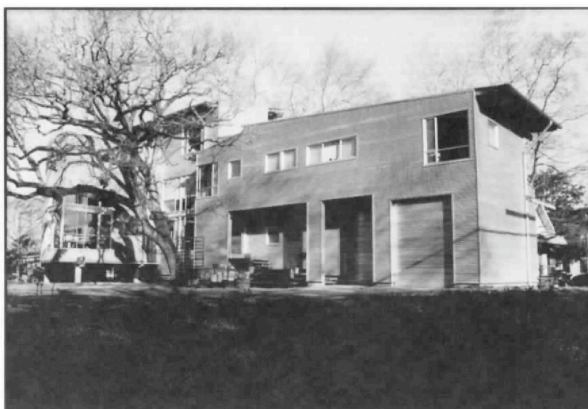
Civitello House, view looking northwest from Asbury street.
