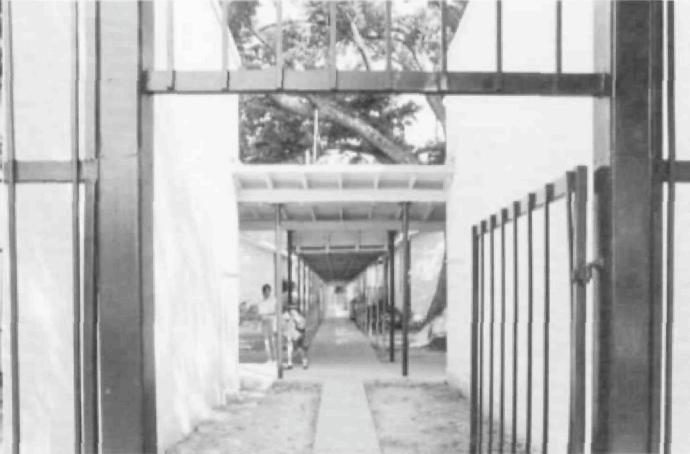
Utilitarian covered walkways to temporary buildings.
