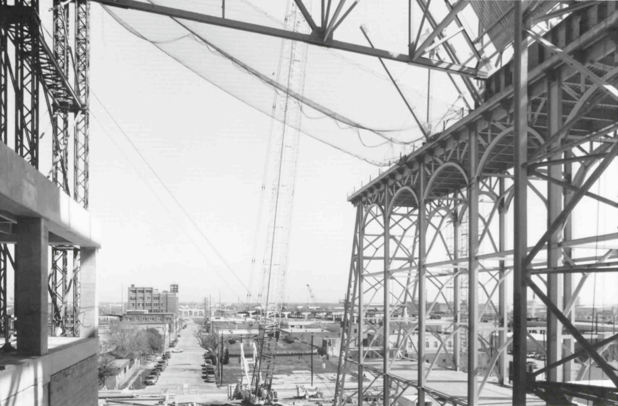
The retro quality of the Ballpark at Union Station's design can already be seen in the arches (right) that will fit beneath the retractable roof.
