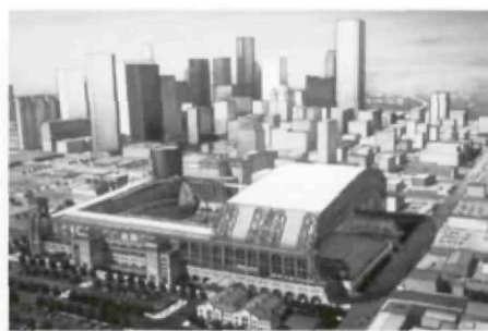
Rendering showing the Ballpark's roof in its retracted state. Fully extended, it would cover the playing field.
