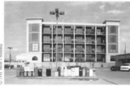
© 1998 Hester + Harshbarger The Metropolis, a Randall Davis loft development at Waugh and West Gray, Page Southerland Page, architect (1997).
