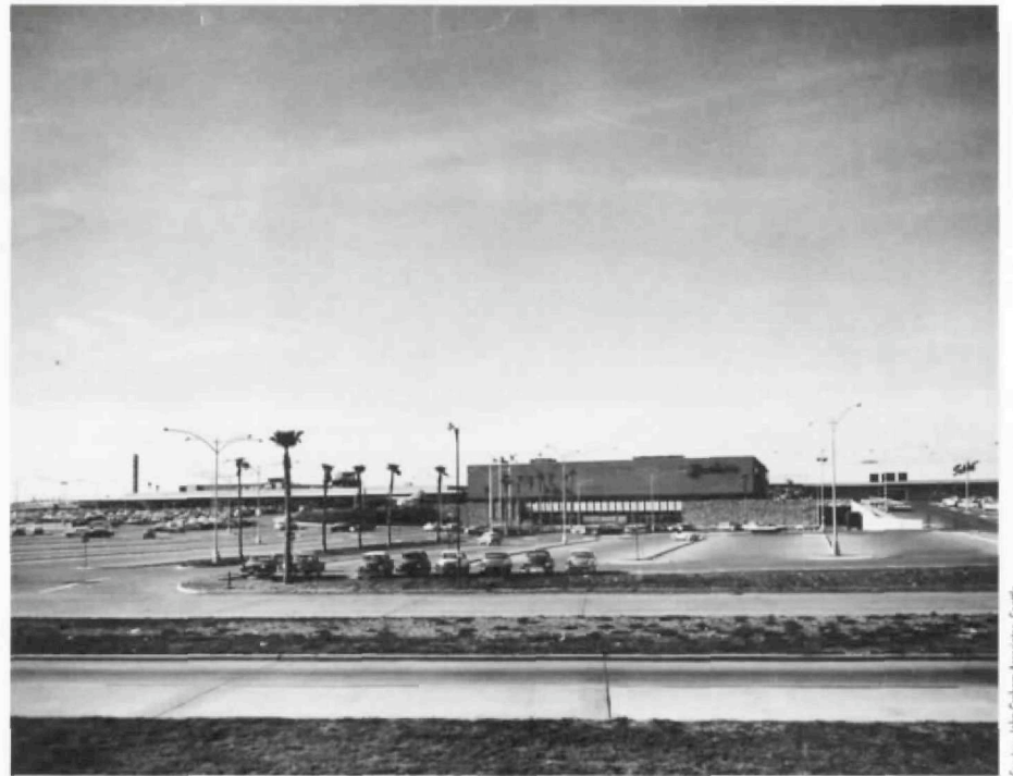
Gulfgate: view from the southeast showing entrance to underground service tunnel on right.
