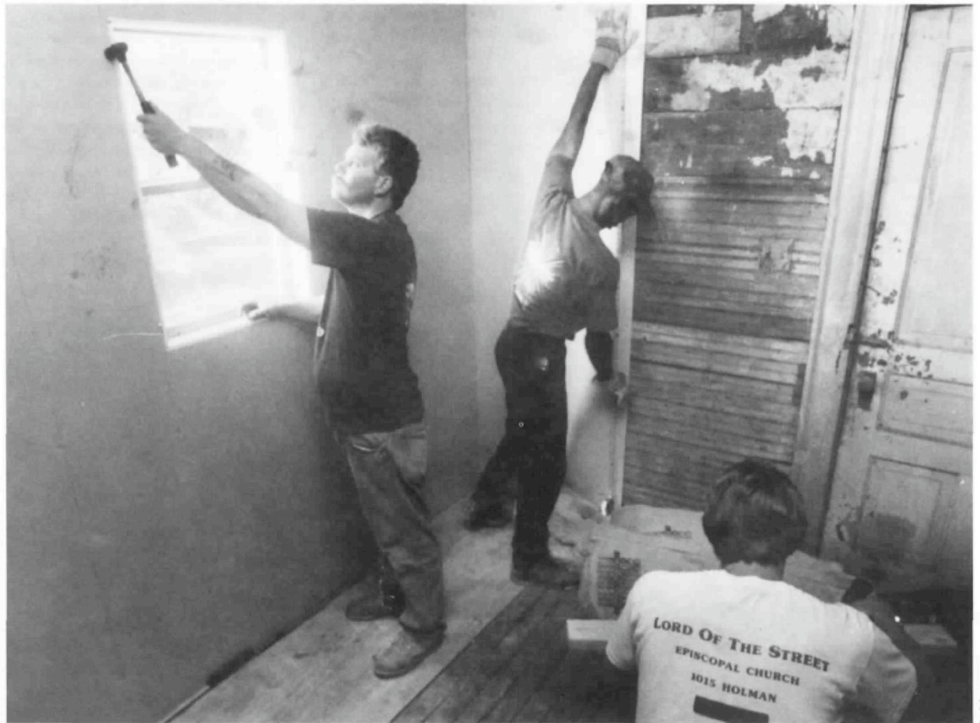
A NOAH crew works on rehabilitating a dilapidated house.
