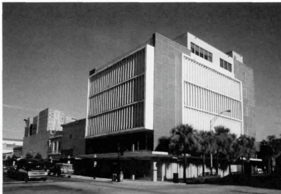
A controversy arose in Savannah, Georgia, about whether to preserve this 1950s Modernist building or refashion it with a more historically compatible façade. The preservation review board rejected the redesign.
