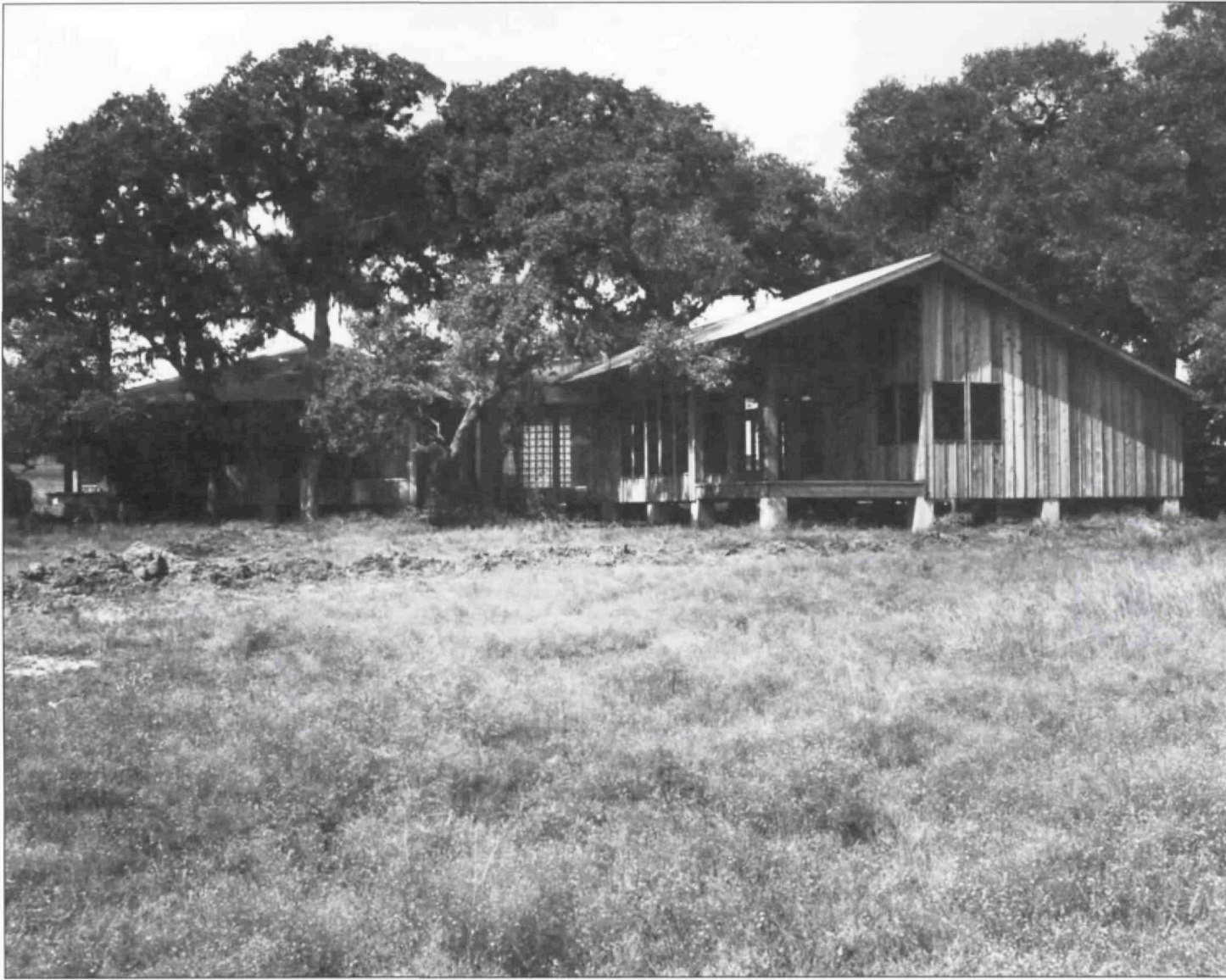
View from the southwest.
