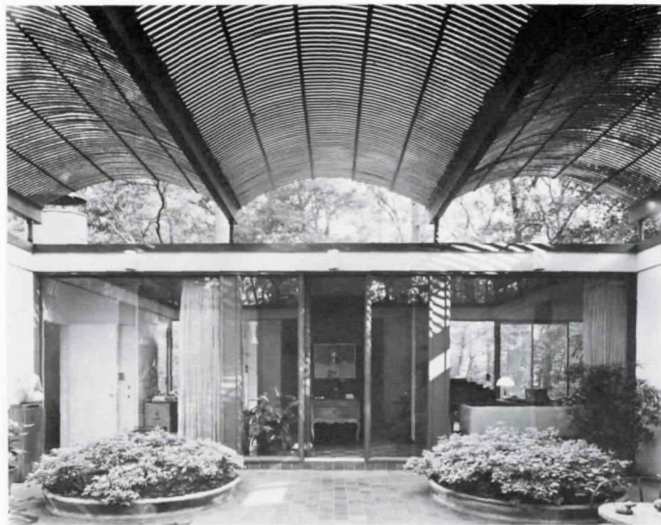
Interior courtyard, Nina Cullinan House, 1953, Cowell and Neuhaus, architects
