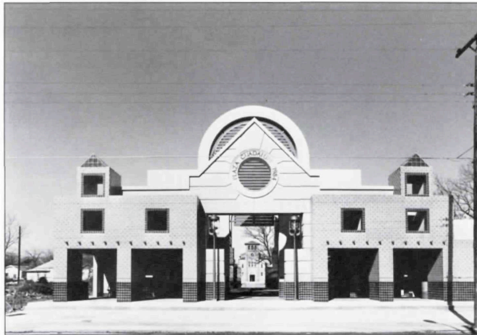
Top: Elevation, Plaza Guadalupe, San Antonio, Reyna Caragone Architects, 1984-89. Guadalupe Street row of storefronts ("Las Tiendas"), phase I.
