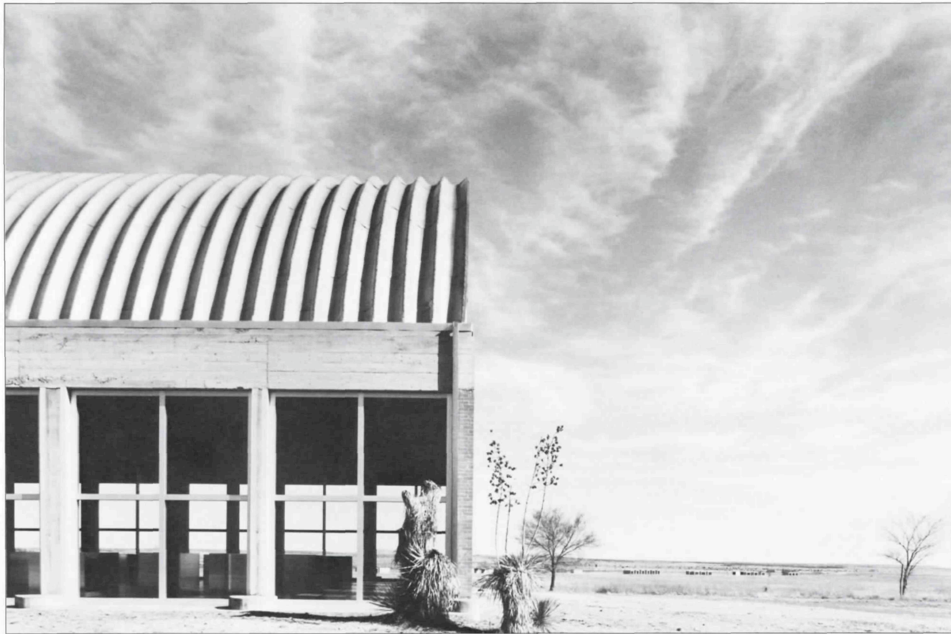
Artillery Shed, Chinati Foundation, Marfa, Texas
