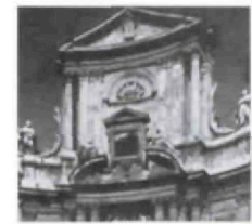
Carlo Fontana, architect, San Marcello al Corso, Rome, detail of upper tier.
