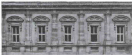
Michelangelo, architect, Farnese Palace, Rome. Detail of court façade, third story, with grouped pilasters.
