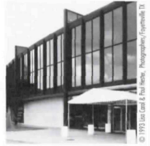
Ludwig Mies Van der Rohe, architect, Museum of Fine Arts, Houston, north entrance with demountable canopy.
