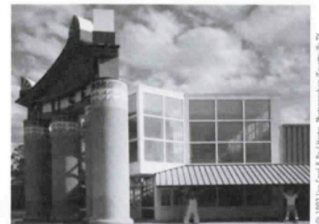
Children's Museum of Houston, perspective view of "portico" and west (parking lot side) elevation.
