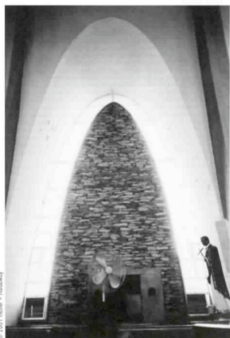
Top and above: Exterior and interior views of the Basilica de la Purísima (1946, Enrique de la Mora and Armando Ravizé Rodríguez).
