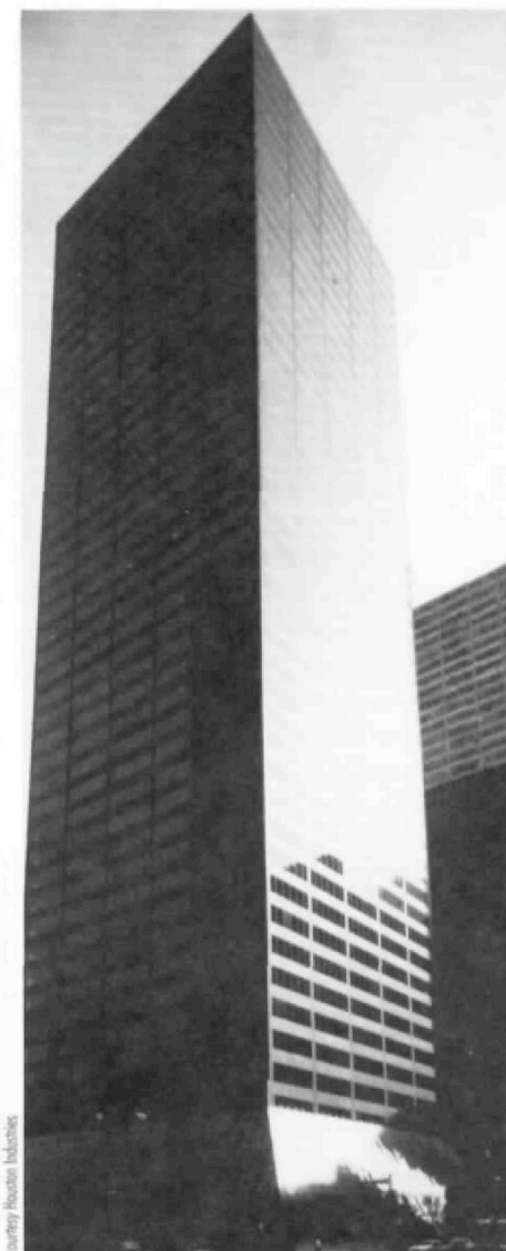
1100 Milam, before renovations, J.V. III, architects, 1973.
