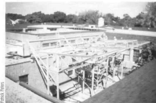
Mechanical Shade Tree under construction.
