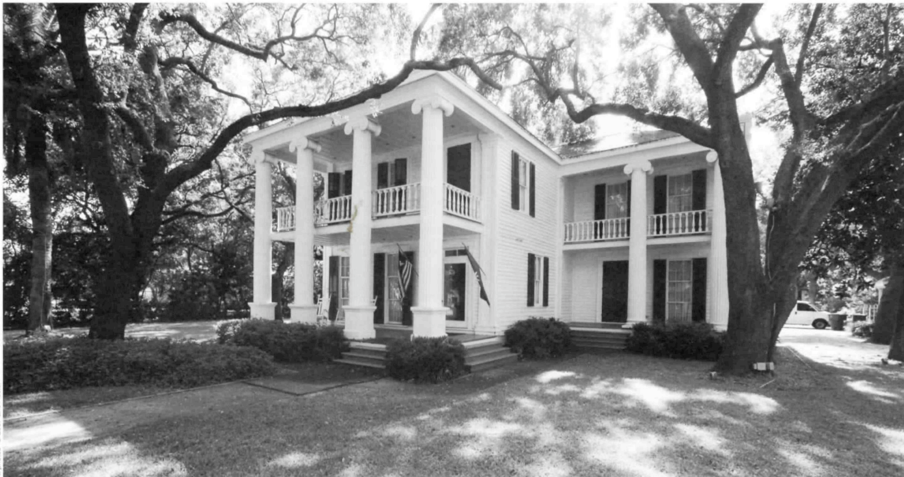
The Michel B. Menard House (1838) in Galveston is a superior Texas example of the Greek Revival approach, with colossal columns and a porch that extends across the façade.
