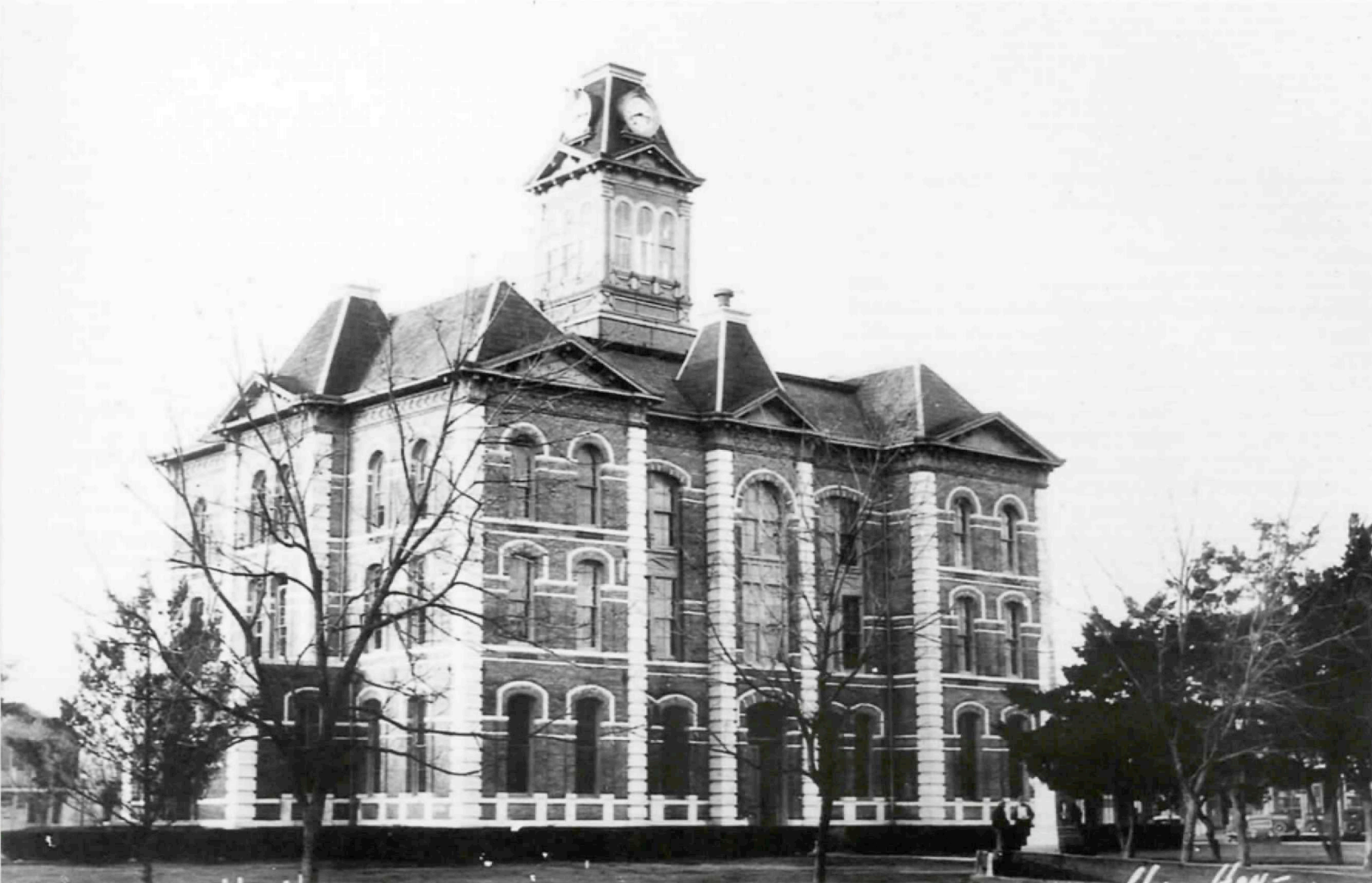
The Wharton County Courthouse as it was: Eugene T. Heiner's 1889 Victorian building.
