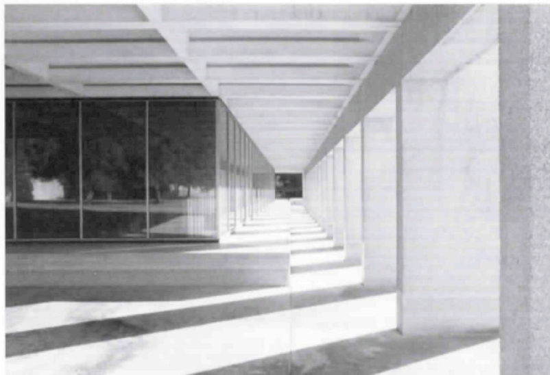
Great Southern Life Building, first floor loggia.
