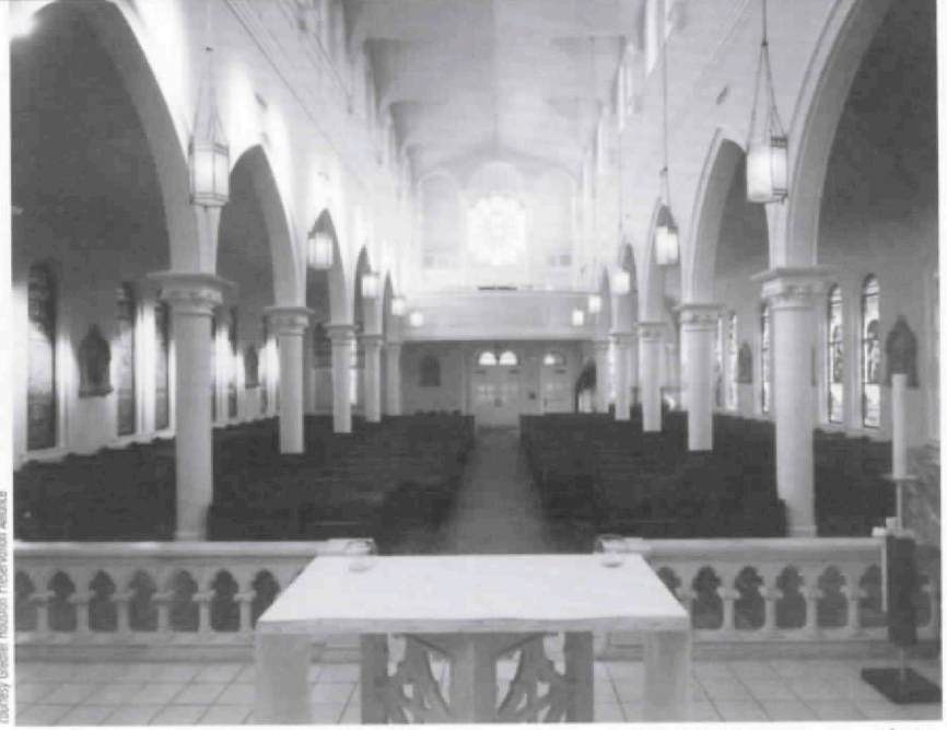
St. Joseph's Church, restored interior; Patrick S. Rabbitt with George E. Dickey, architects, 1901. Restoration team: John J. Dasek, AIA, architect; Leslie Barry Davidson, AIA, interiors consultant.
