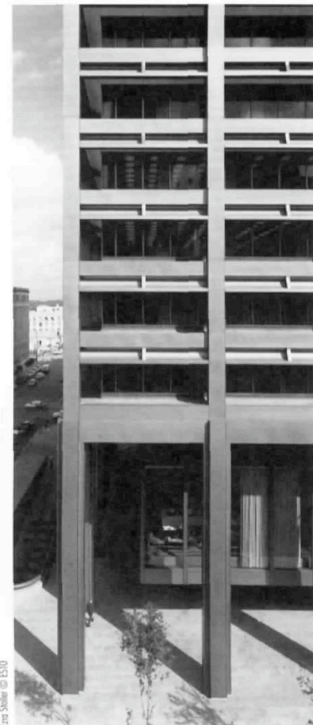
Tenneco Building, corner at ground level with garage entrance at left.
