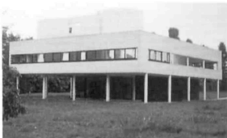
Villa Savoye, outside of Paris, France, Le Corbusier, architect, 1928-30.
