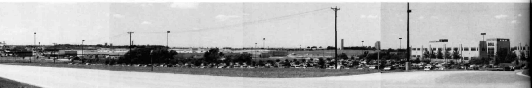
Dell Plant, Austin. Photos © 1997 Hester + Hardaway
