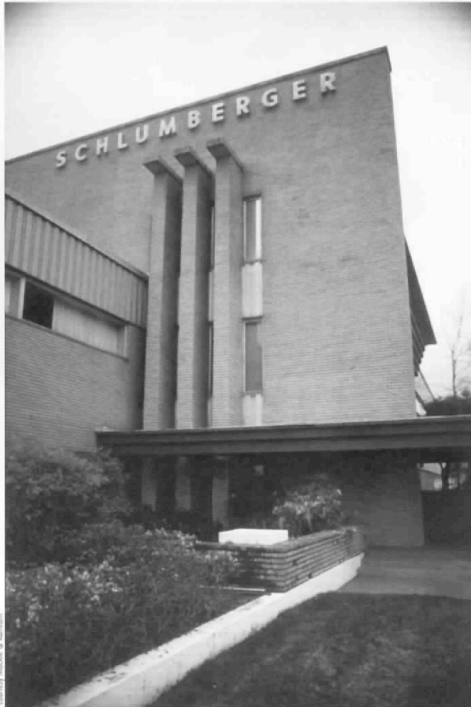
Schlumberger Well Services Headquarters, 5000 Gulf Freeway, MacKie & Kamrath, architects, 1953.
