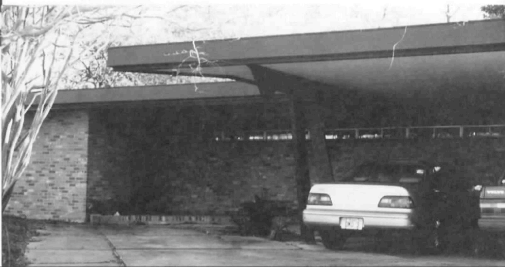
3611 N. Braeswood Boulevard, Herb Greene with Joseph Krakower, architects, 1957.
